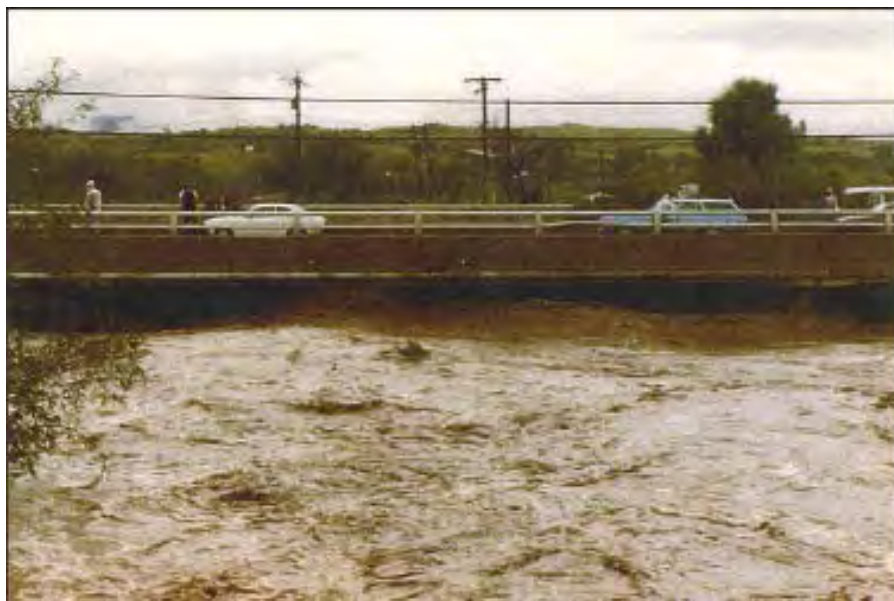
Figure 3 – Highway 82, Sonoita Creek, Oct 1983
